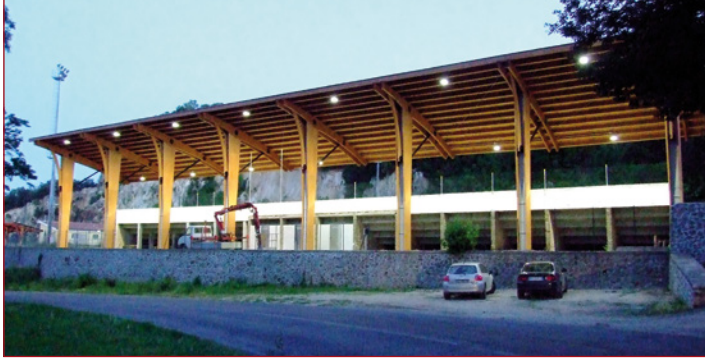
Laminated wood structures with integrated photovoltaic systems implemented in the municipalities of Santa Marinella and Allumiere (Rm) as a result of a program agreement drawn up between Enel Green Power and Municipal Authorities.
